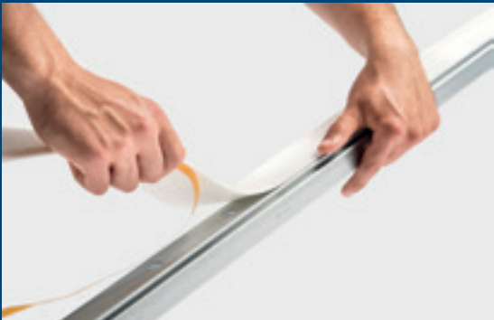
↑ Anchor Geberit Duofix system rails on the floor and ceiling. Attach the Geberit Duofix acoustic insulation tape and anchor the system rails in the floor and ceiling.
