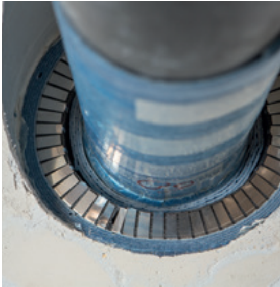
↑ Professional installation of a discharge pipe in an oblique ceiling opening. A fire protection sleeve is located between the pipe and the concrete.
